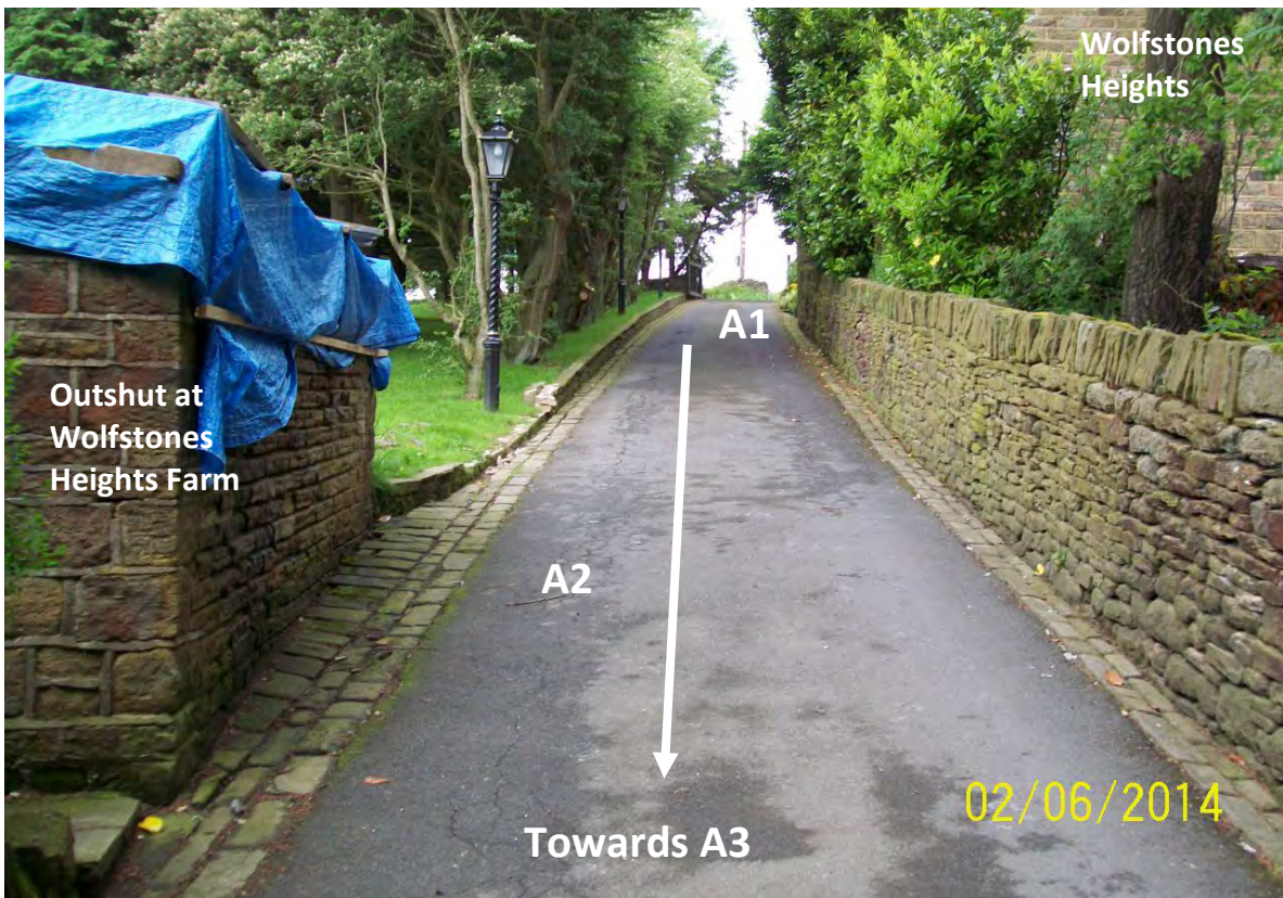
14. View west from near point A2 towards point A at Wolfstones Road. To the left (south) is an outshut forming part of Wolfstones Heights Farm. This part of the building had been damaged by fire in December 2013. 02 Jun 2014.
